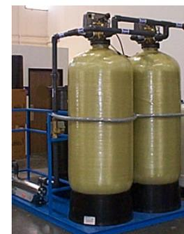
Systems Shown with Optional Skid Mounting and Control Panel
