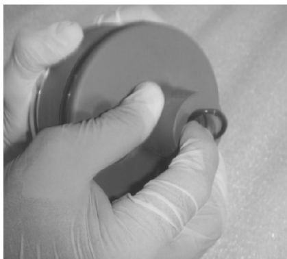
Installing PWT Seal
