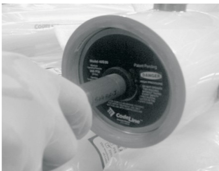
Installation of the End Plug Assembly into the vessel
