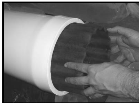
Installing thrust ring
