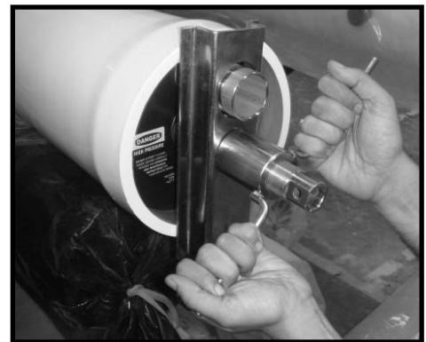
Removing Head Assembly using Head Tool
